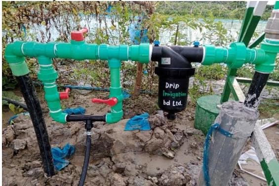
Mainline, DIBL Filter and venture setup
