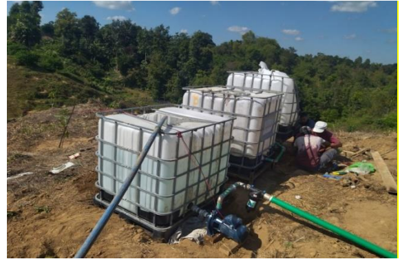
Mainline Pipe networking and Tank Setup
