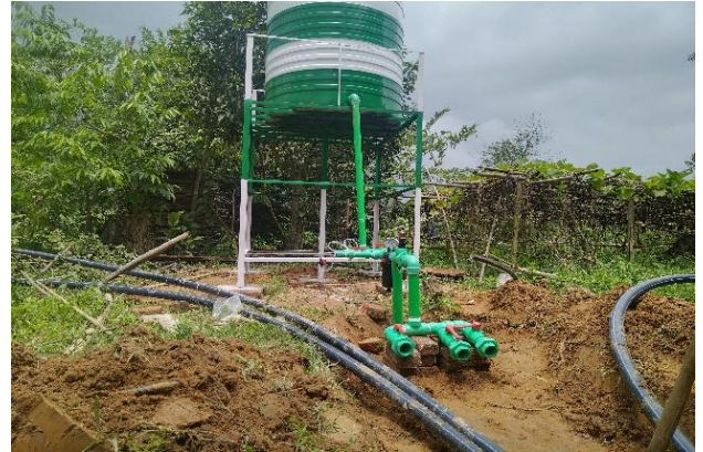
Main line joining with Tank
