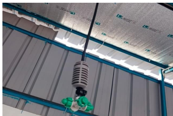
Water discharge by dripper nozzle
