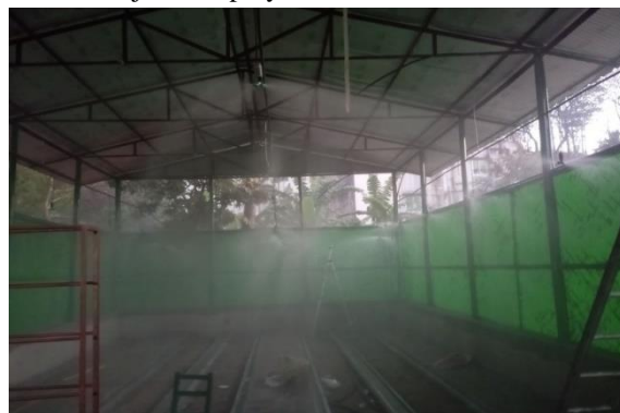
Water discharge by fogger nozzle
