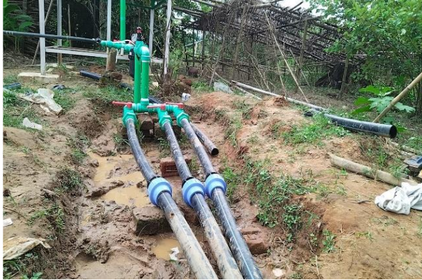
Mainline Irrigation setup from water pump
