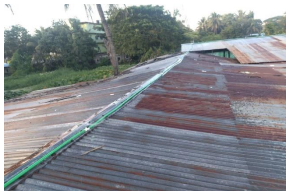
Sprinkler setup above shed
