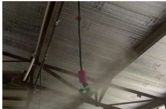
Water discharge by dripper nozzle
