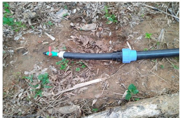
Flash Valve setup in the mainline ending point
