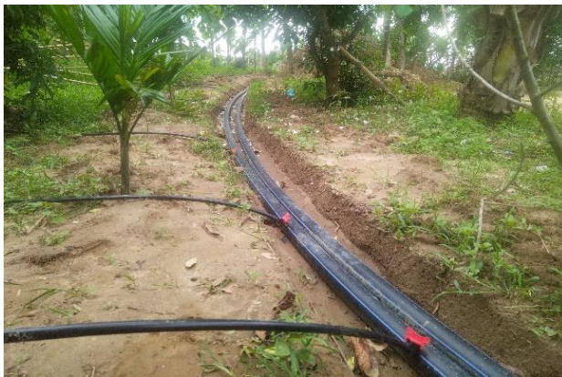
16mm tube with bypass connector in mainline
