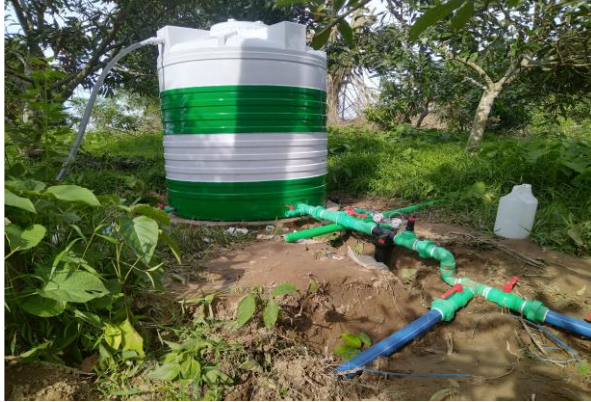
Mainline Irrigation Setup From Tank
