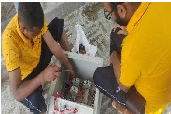
Automation DB BOX Setup
