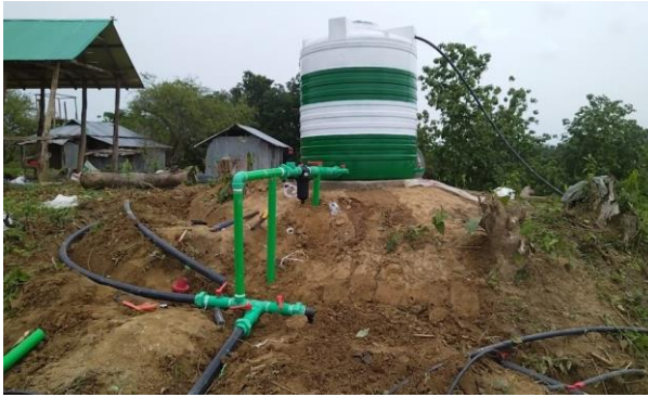
Mainline Irrigation Setup from Tank
