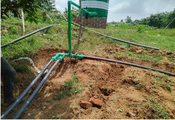
Mainline Irrigation setup from Tank
