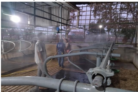
Fogging system running
