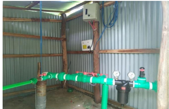
Pump, Filter and pipe setup
